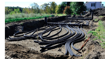
Figure 2 Laying out the first of three layers of heat exchange tubing.
