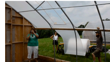
Figure 1 Installing Solawrap on a high tunnel, one 4 foot plastic panel at a time. Each panel is secured to the high tunnel frame.
