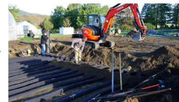
Figure 3: Backfilling soil onto the last layer of the heat exchange tubing. This last layer must be at least 12 inches below the soil surface.
