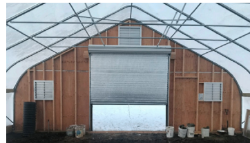
Figure 5: Inside the climate battery, newly installed just in time before the snow. Notice the black air intake riser to the left (before mylar ducting is attached to draw warm air from higher up in the high tunnel).
