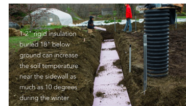
Figure 4: Installing the rigid insulation after the underground climate battery installation is complete.
